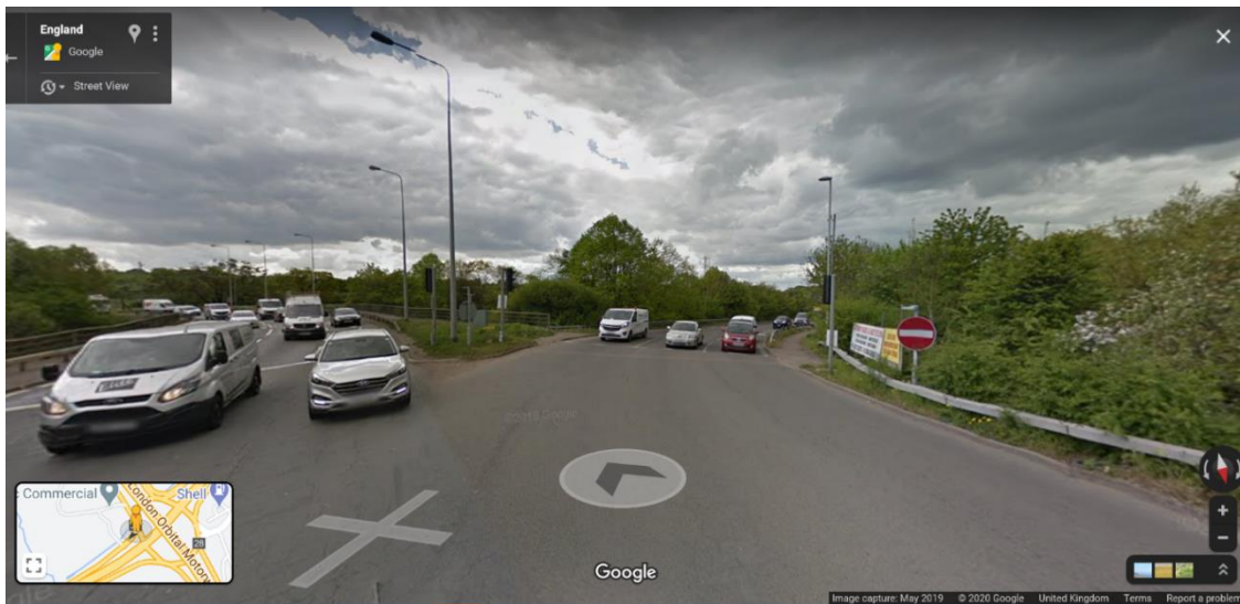
FIGURES 21, 22 AND 23 BROOK STREET INTERCHANGE
